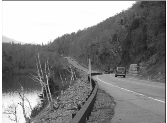
Cascade Notch, one of the areas ecologically damaged by large amounts of road salt.
