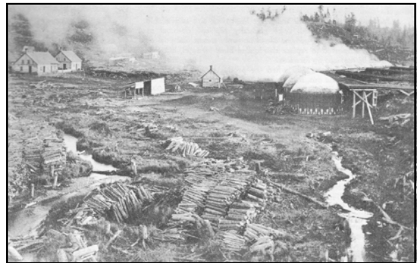
Charcoal Kilns constructed to supply fuel to Iron Forges and Bloomerys. Similar Kilns once sat on the banks of the Ausable River near Church Street, Keene. Photo from McMartin, 1994.
