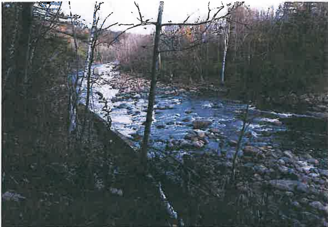
Photo 9 Dam ID# 219-1082 Rome Dam 10/22/13 Outlet channel
