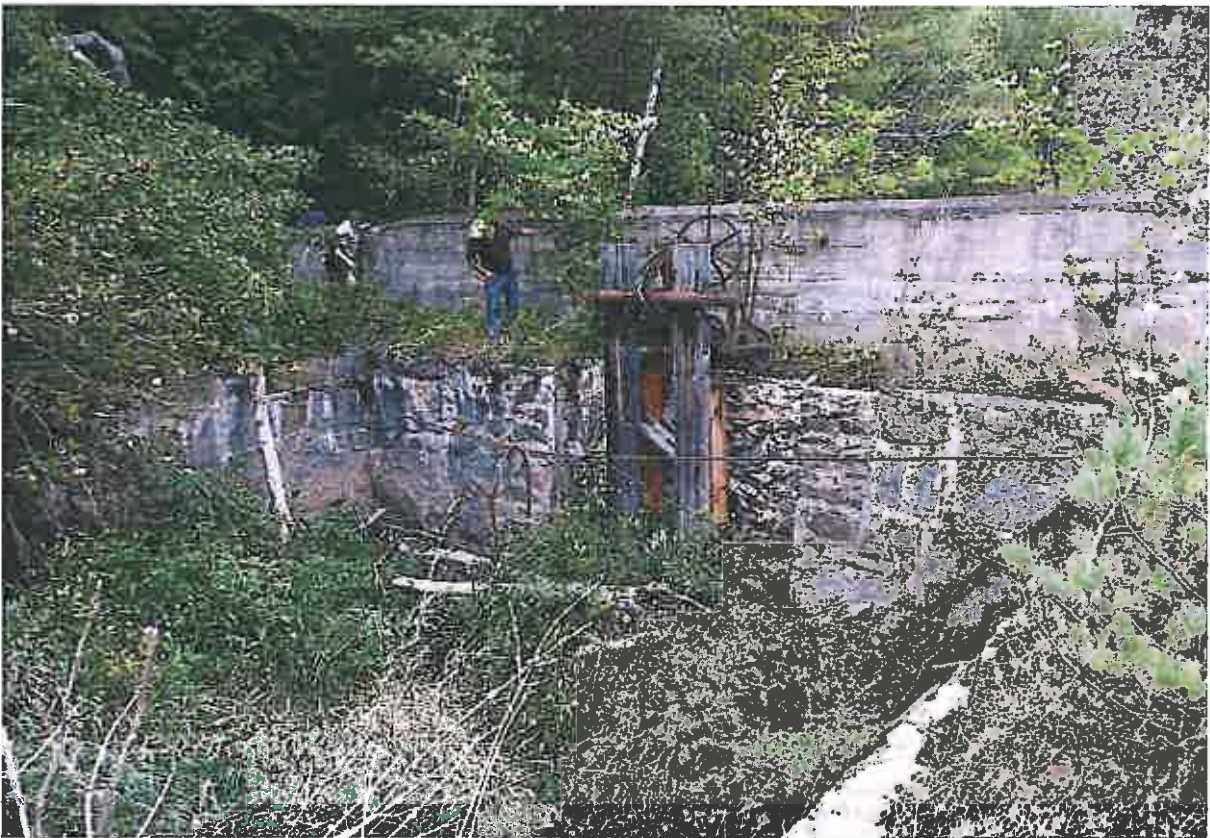
Photo 10 Dam ID# 219-1082 Rome Dam 9/14/15 Left penstock intake
