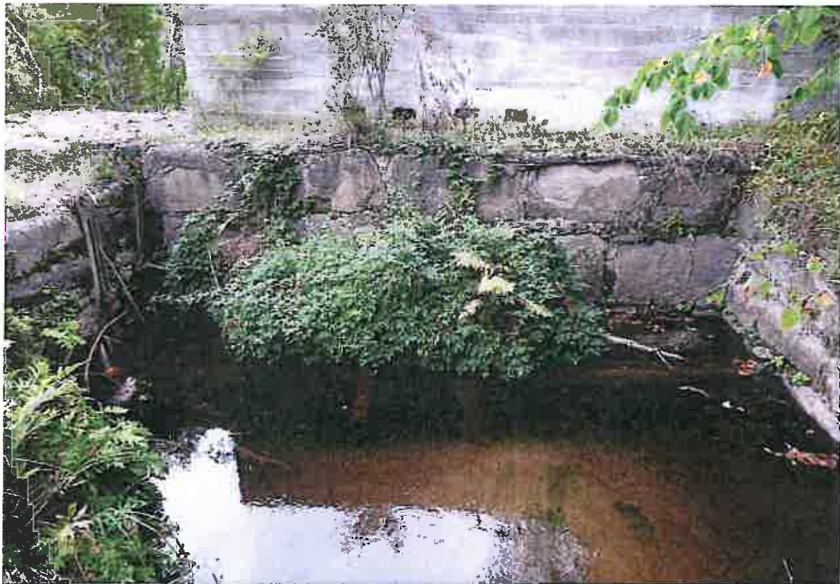
Photo 4 Dam ID# 219-1082 Rome Dam 9/14/15 Right penstock intake
