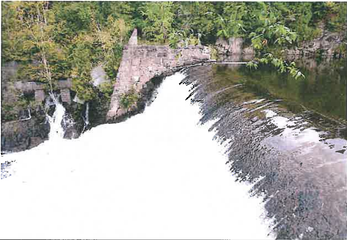
Photo 9 Dam ID# 219-1082 Rome Dam 9/14/15 Looking east across spillway
