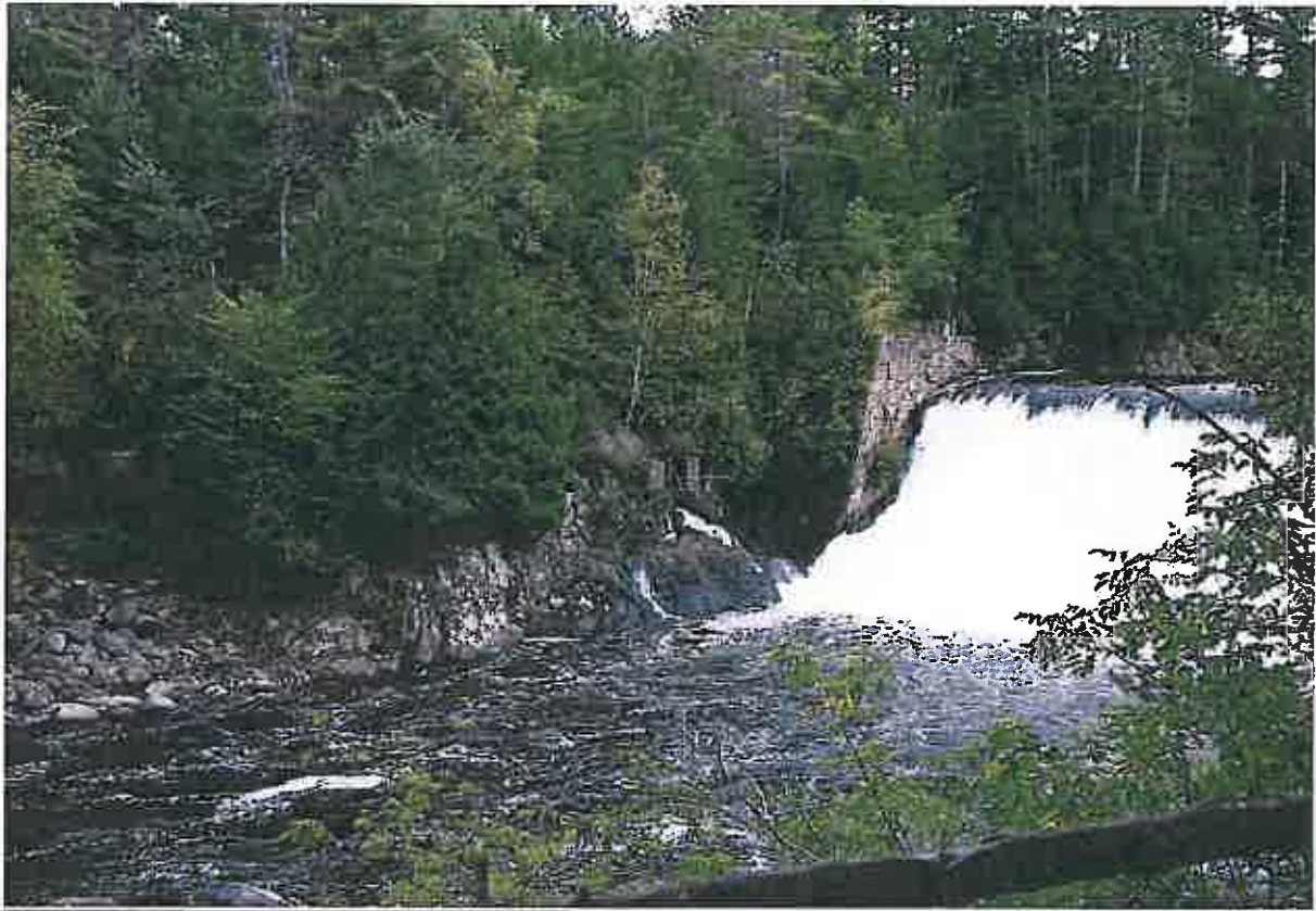
Photo 5 Dam ID# 219-1082 Rome Dam 9/14/15 Looking southeast at right abutment, penstock
