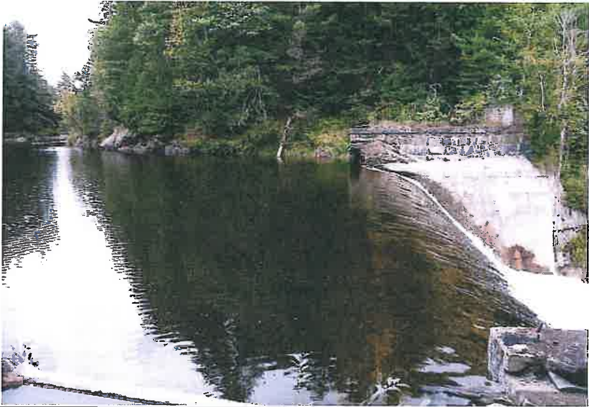
Photo 1 Dam ID# 219-1082 Rome Dam 9/15/15 Looking west across spillway
