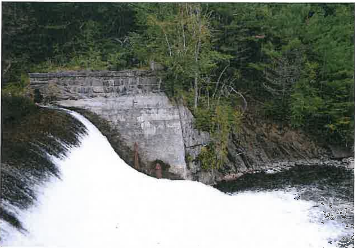
Photo 3 Dam ID# 219-1082 Rome Dam 9/14/15 Left spillway sidewall
