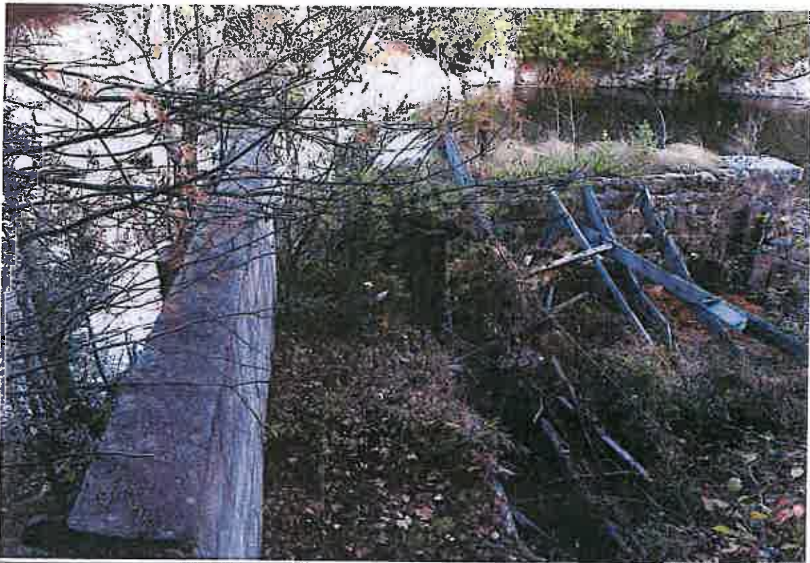
Photo 7 Dam ID# 219-1082 Rome Dam 10/22/13 Looking across left intake from bank
