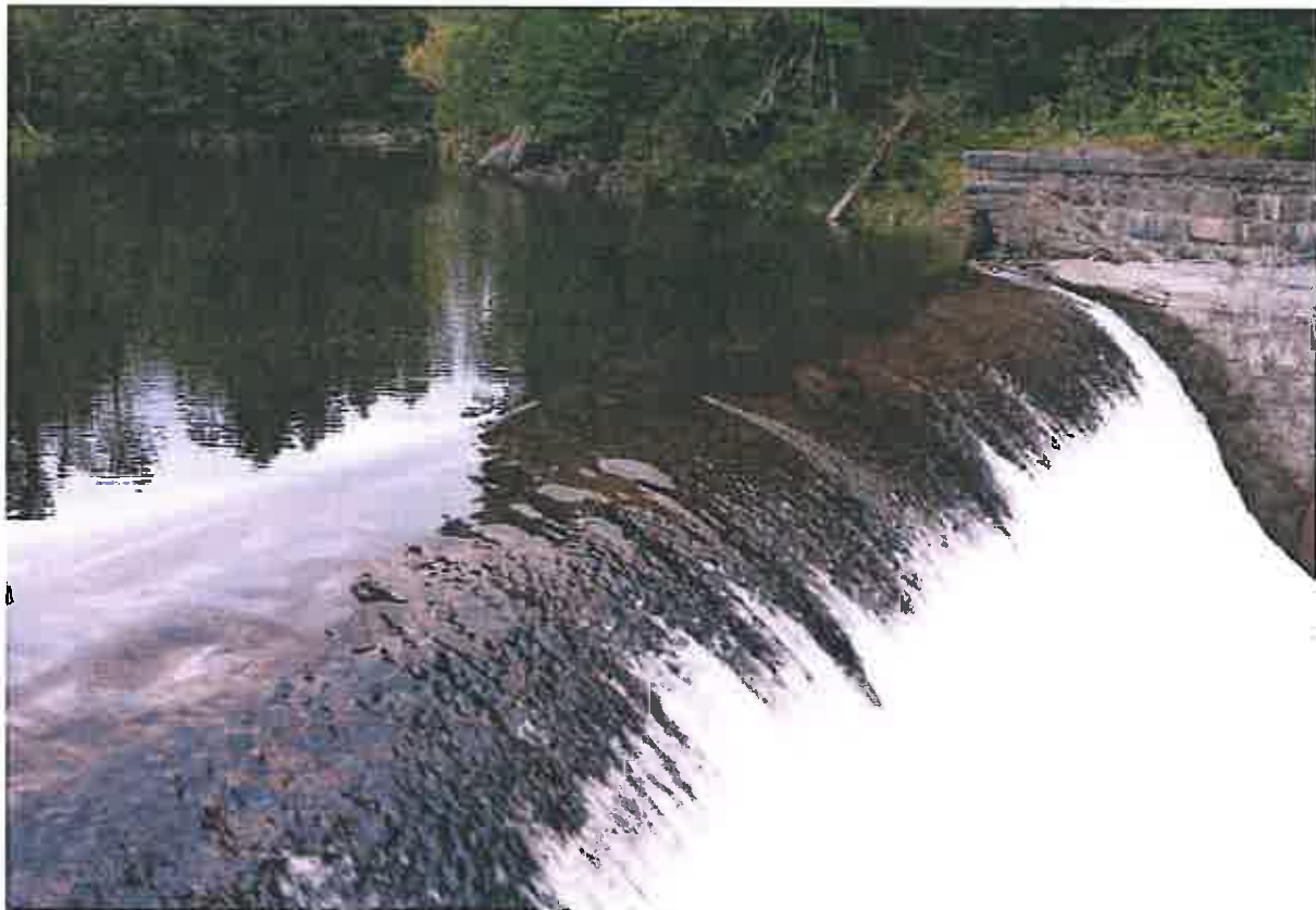
Photo 2 Dam ID# 219-1082 Rome Dam 9/14/15 Spillway crest
