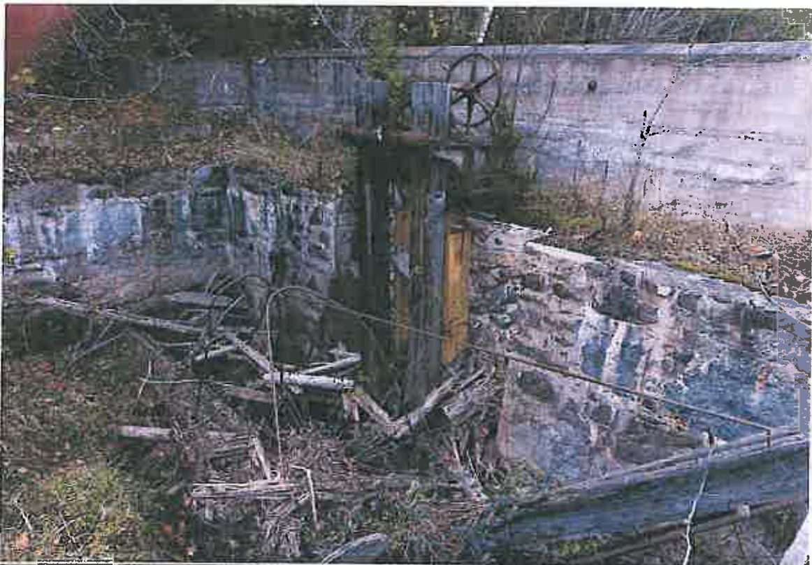
Photo 5 Dam ID# 219-1082 Rome Dam 10/22/13 Left gate, intake structure
